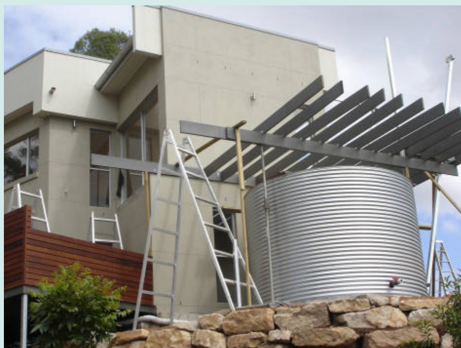
Multiple rainwater tanks are attached to each house at the Payne Rd development (The Gap, Brisbane). There are also three communal rainwater tanks.
